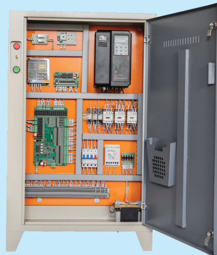
V3F (Variable Voltage, Variable Frequency Micro Processor Control-Jerkless Travel
